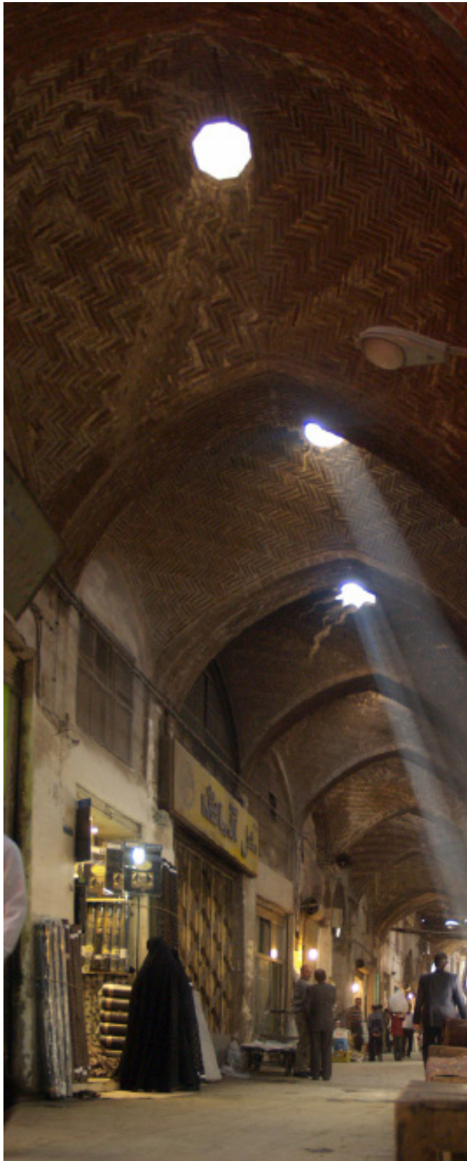
Bazar-e Bozorg, Isfahan, October 2007. The herringbone bond of the masonry domes gives the structure an almost woven quality. This is in the northernmost, poorer part of the long bazaar. The bazaar consists of several covered streets, the longest of which connects imam square with the friday mosque 1½ winding kilometers away (seier+seier, Flickr.com).
